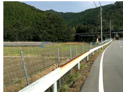
Fence along the Road
